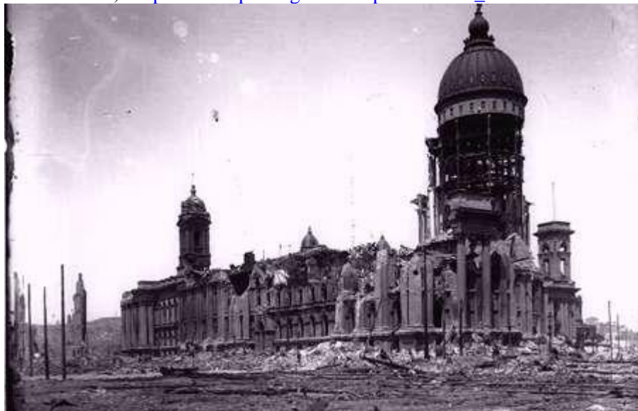
San Francisco City Hall after the 1906 Earthquake. (from Steinbrugge Collection of the UC Berkeley Earthquake Engineering Research Center)
