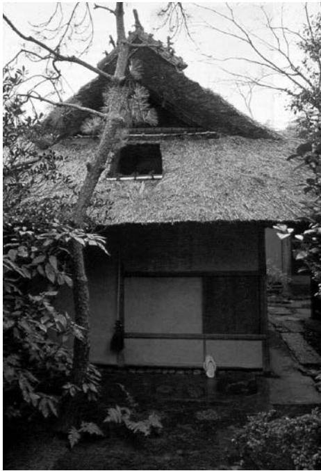
Exterior view of Yuin tearoom [Urasenke Konnichian], early 17th c. Built for Sen Sotan in the taste of Rikyu.
